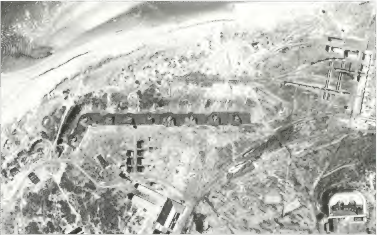
Figure 5.43. Aerial photograph of Nine Gun Battery, January 1933. This photograph shows the engineered slope of Nine Gun Battery with limited vegetation. To protect the earthwork, all woody vegetation greater than four-inches diameter at breast height should selectively removed. The area north of Battery Alexander appears darker in this image because it is the north slope and in shadows (Coastal and Hydraulics Laboratory, Engineer Research and Development Center).
